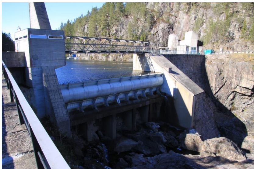
Figure 4-2: Gated Spillway in Vrangfoss Dam
