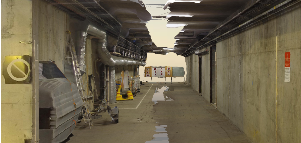
Figure 4.6: 3D mesh model produced from photos captured with GoPro provided by Context Capture
