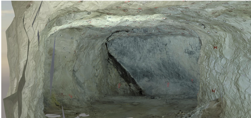
Figure 5.16: The inside view of the second model in Drift A
