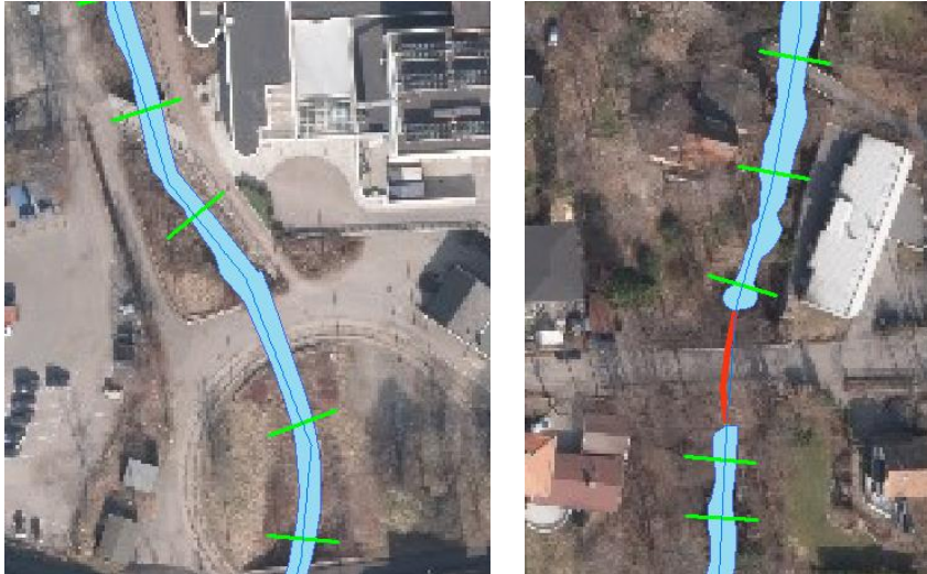
Figure 52: Examples of neglected culverts
