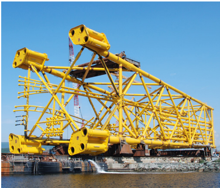
Figure 2.10: Jacket Gudrun load-out, Kvaerner (2015)
