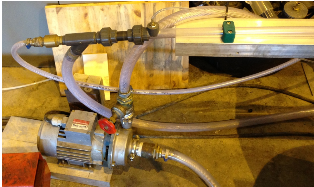
Figure C.3: A close up view of the pump, the pipe inlet with both gas and liquid inlets and the foam generator
