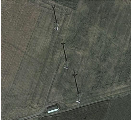
Figure 2: Top view of the wind farm
