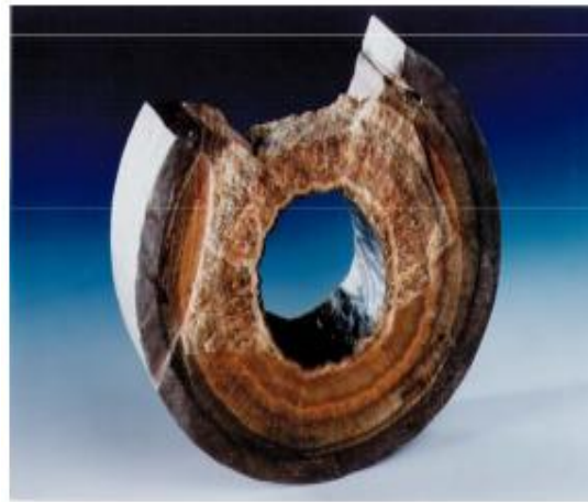
Figure 17: Scale deposits on a pipe's section (Time 2011).
