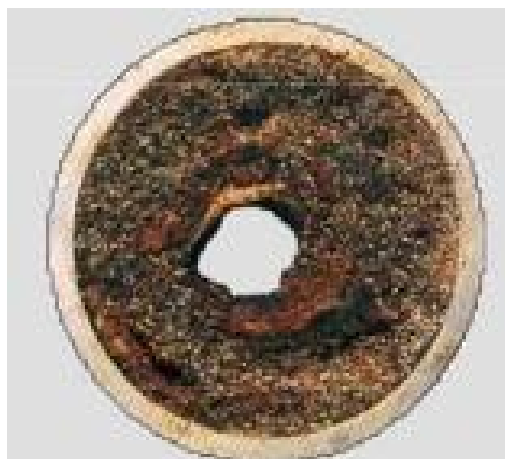
Figure 14: Wax deposits on a pipe's section (Time 2011)
