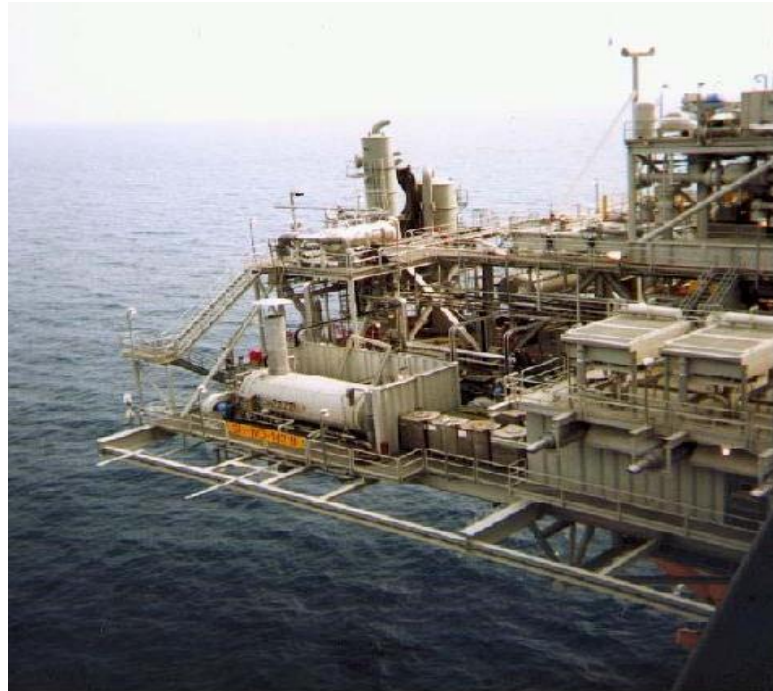
Figure 23: Photograph of Glycol Regeneration & Reclamation Unit (Son and Wallace 2000).
