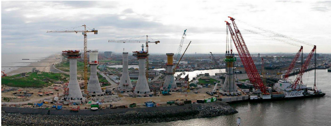
Figure 4.11: GBS under construction in Belgium, Thornton Bank Project [1]
