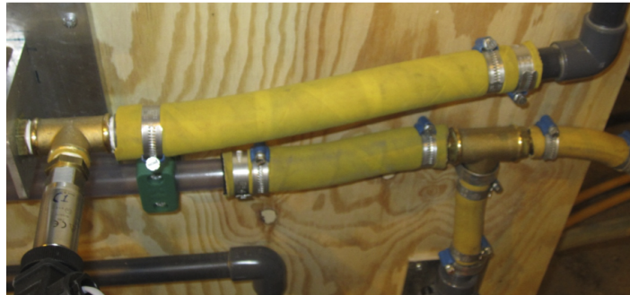
Figure 5.1: Hose parts and pipe clamps on control board.
