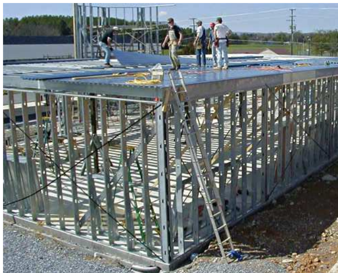
Figure 30: Steel bearing wall system
