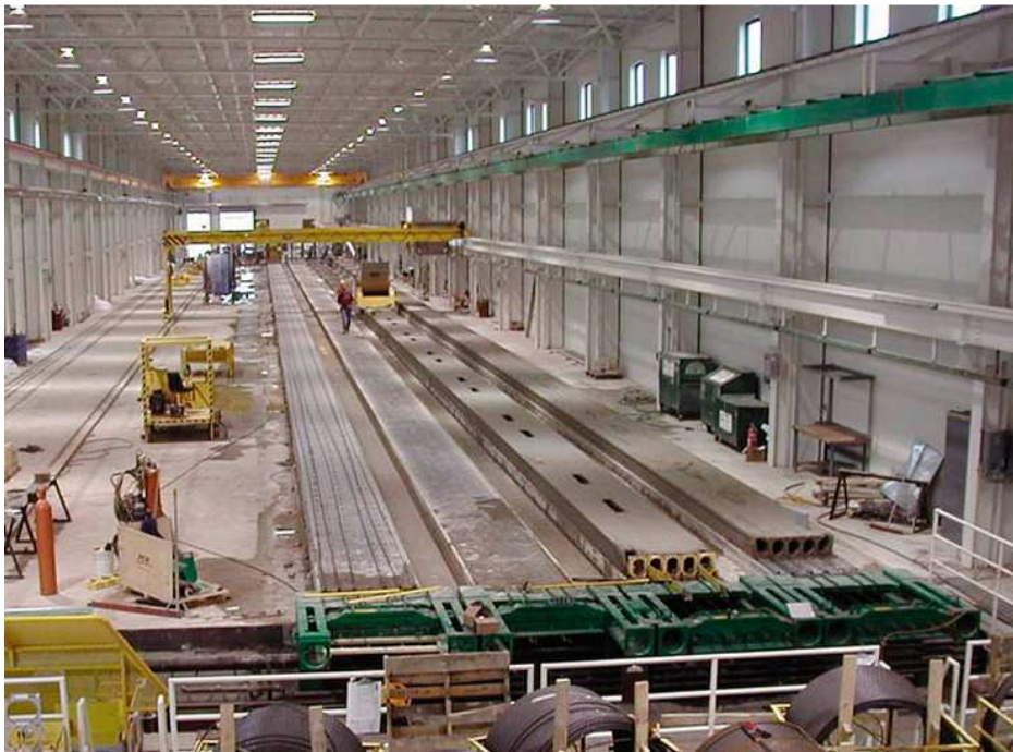
Figure 38: Interior of a general prefabrication plant
