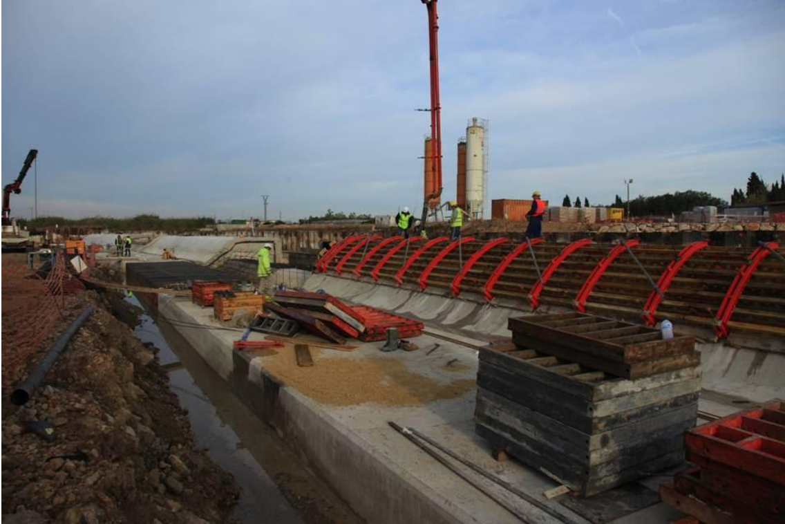
Illustration 28: Building the azud
