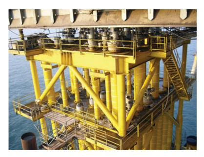
Figure 1.3: The picture shows the cellar deck. Notice the x-mas trees placed on the top deck with the risers continuing down towards the sea (Fu et al., 2009).
