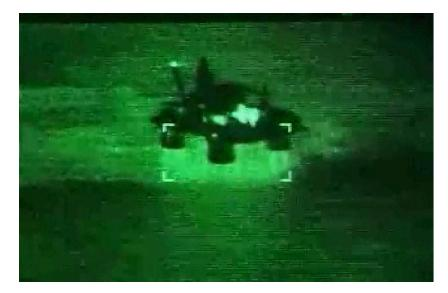
Figure 4.9: The picture taken by a night vision camera on board one of the helicopters approximately at 2 a.m. captures the heat of the gas underneath the rig (Statoil, 2005).
