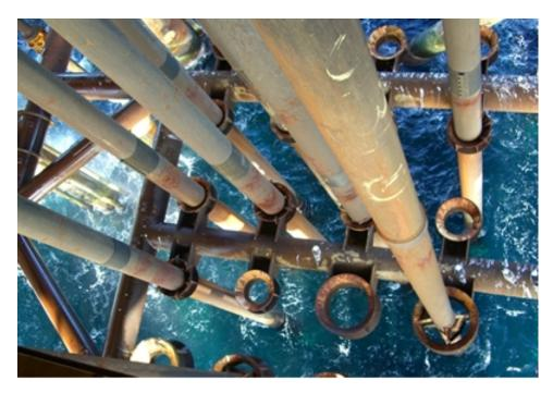
Figure 1.2: The figure shows how a slot layout on a platform looks like. Note that there are several free slots on this platform (Claxton, 2012).
