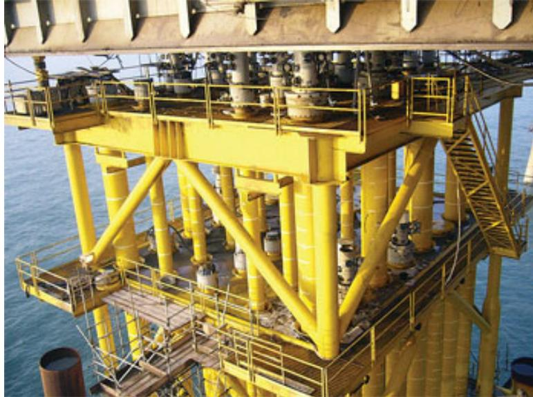
**Figure 1.3:** The picture shows the cellar deck. Notice the x-mas trees placed on the top deck with the risers continuing down towards the sea (Fu et al., 2009).
