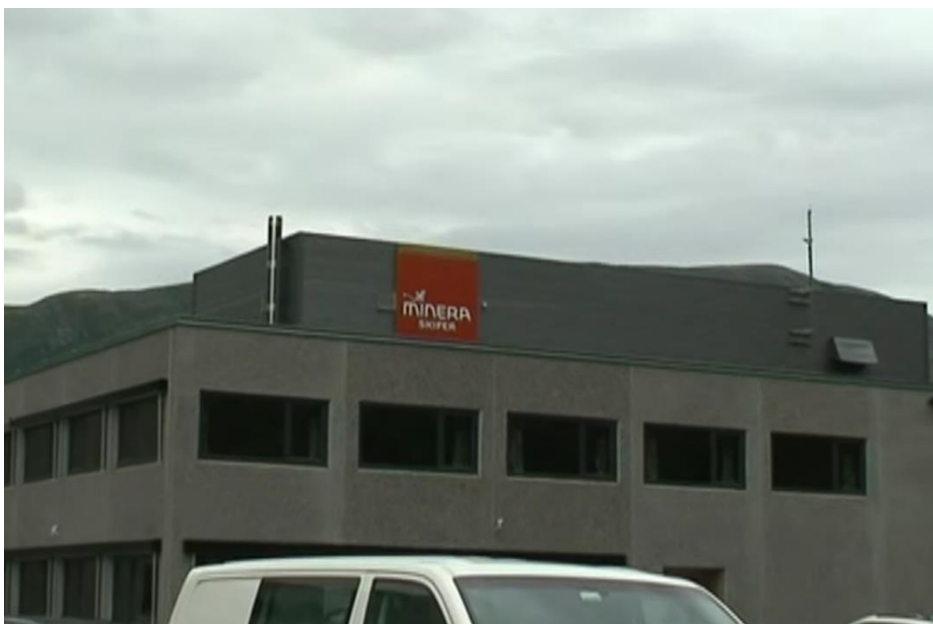
Figure 6.1 Minera Skifer plant in Oppdal
