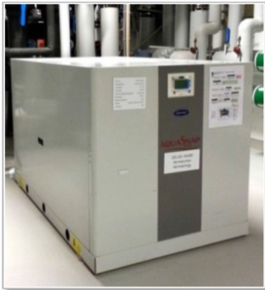
Figure 25 The heat pump and liquid chiller unit at Powerhouse Kjørbo for space heating, heating of ventilation air, and back-up space cooling (Nordang, 2014/15).
