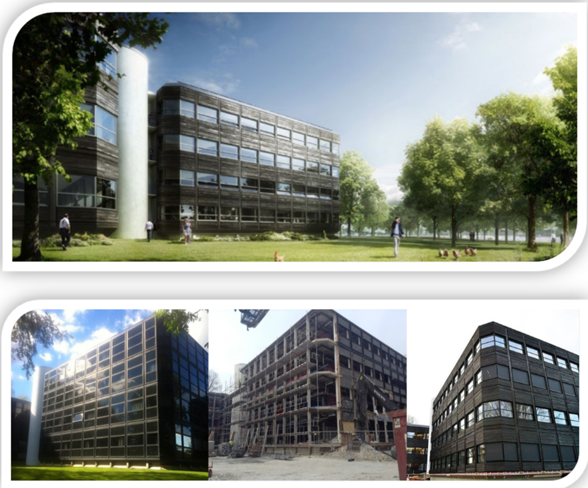
Figure 23 Powerhouse Kjørbo – a 5,200 m 2 office building in Sandvika refurbished and upgraded to passive house standard. The building was BREEAM-Nor certified as "Outstanding".
