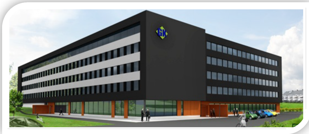
Figure 14 Miljøhuset GK – a 13,650\text{ m}^2 office building in Oslo of passive house standard. The building was certified as "Very good" according to the BREEAM-Nor classification system.
