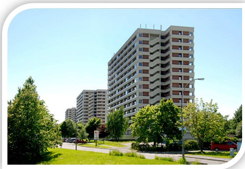
Figure 1 Three block of flats at Tveita Borettslag (housing cooperative) with totally 819 flats.
