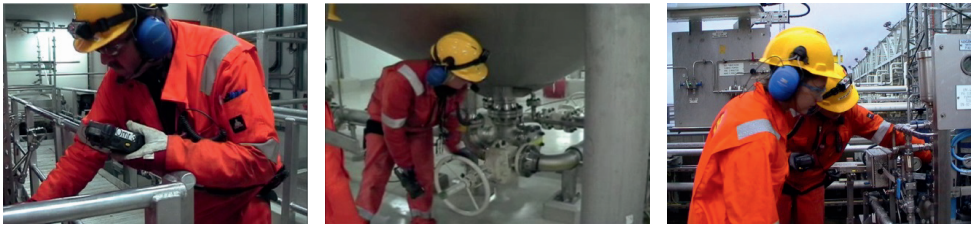
Figure 6-7: Operators performing data logging mediated by a handheld PDA. During the logging procedure, operators will perform other operations that will not require the PDA. These operations can either relate to the same action (e.g. maintenance work as part of plant operation) or to another action (e.g. signing of work permits as part of administration).
