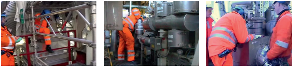
Figure 3-11: User tasks: In industrial process facilities, such as in the oil and gas industry, a typical activity of an operator often is to get from point A to point B. A primary task thus becomes to navigate through a network of pipes and valves, whereas the operation of a mobile device becomes a secondary task (Photographs: author).
