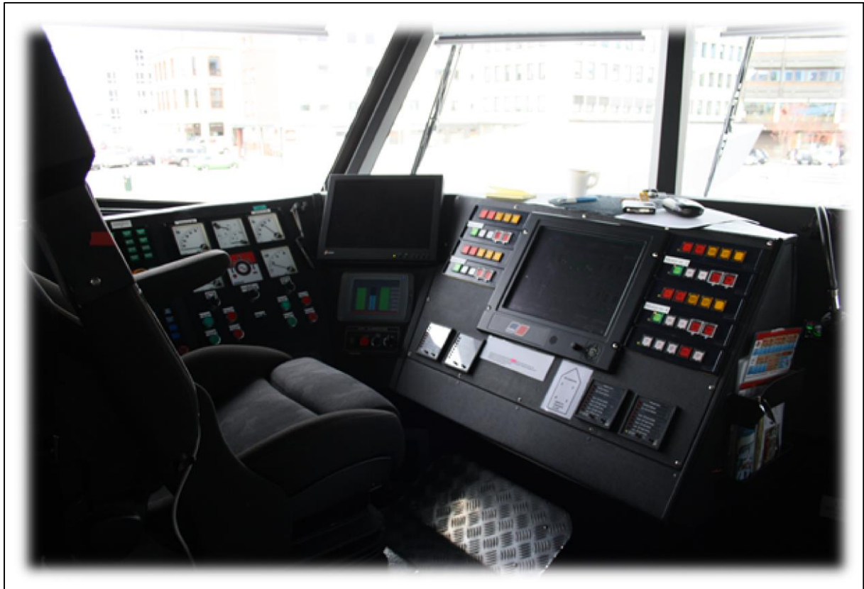
Figur 2-14 Chief engineers place on bridge (Åfeldt Jimmy).
