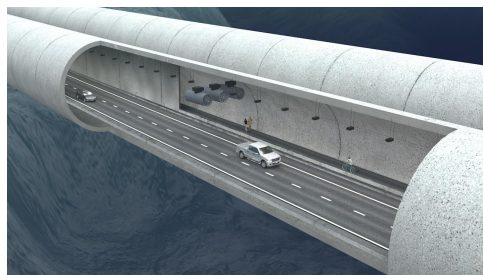
Cross-section of submerged floating tunnel 2
