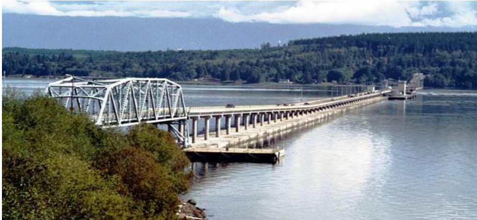
Figure 3: Hood Canal Bridge [6]
