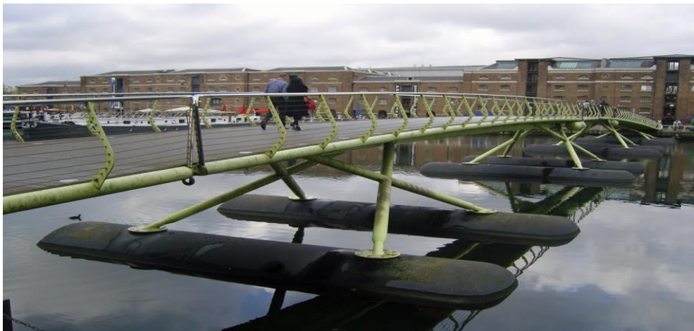
Figure 10: West India Quay Floating Footbridge [14]
