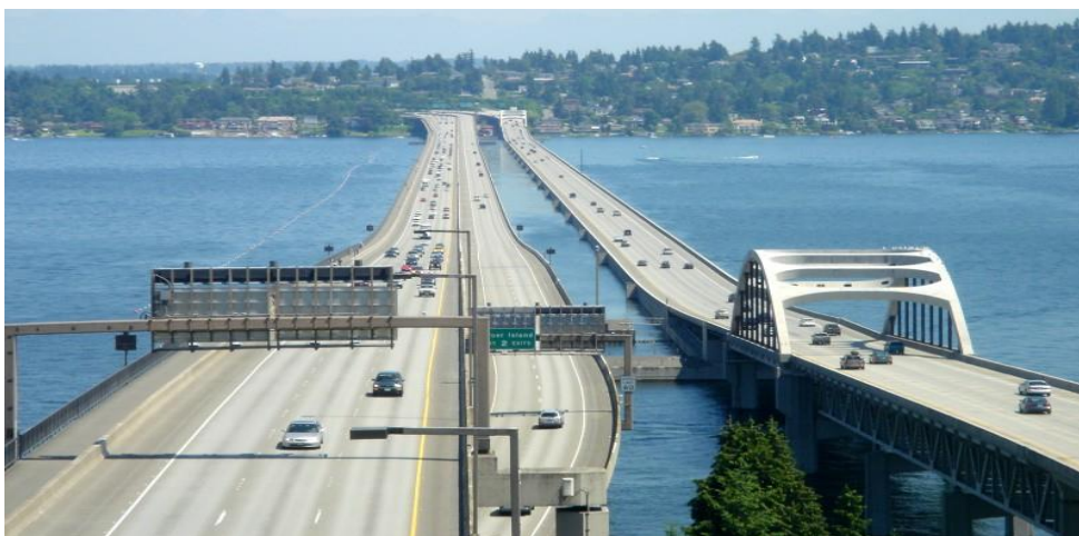
Figure 2: Homer Hadley Bridge (left) and Lacey V. Murrow Memorial Bridge (right) [5]
