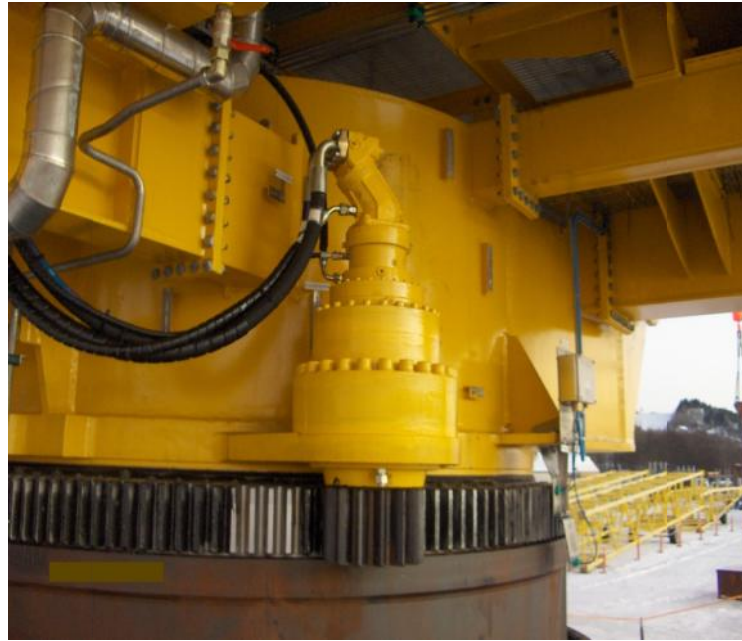
Figure 7: Slewing ring in the crane in practice
