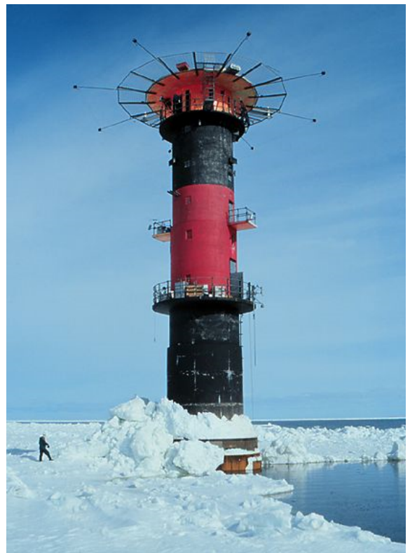
Figure 2.5: Norströmsgrund lighthouse. Photo courtesy of LTU.
