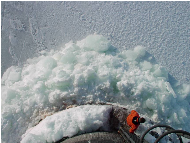
Figure 2.1: Ice crushing against the Norströmsgrund lighthouse. Photo courtesy of Kari Kolari.
