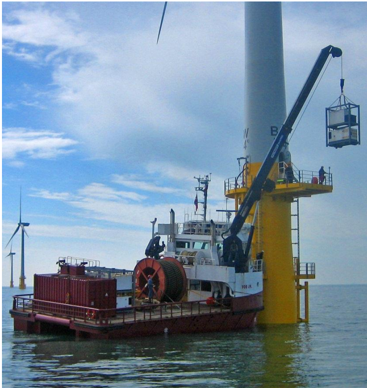
Figure 2.5 - Light crane operation on an offshore wind turbine (32)
