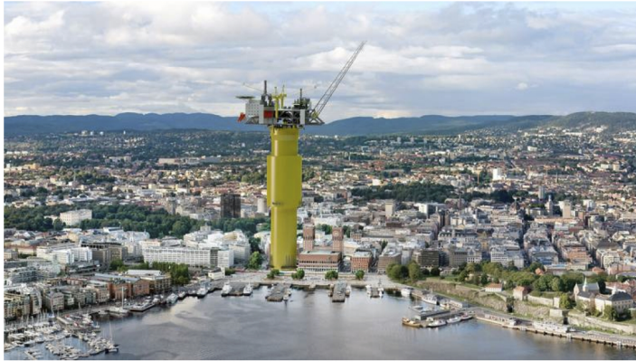
Figure 1.1: Aker Solutions idea of a SPAR platform with a stepped cylinder design producing oil at a record depth of 1300 meters. To give an impression of its size the platform is compared against high-rise buildings in Oslo. Reprinted from www.aftenposten.no , PHOTO: Aker Solutions/Giga pix AS
