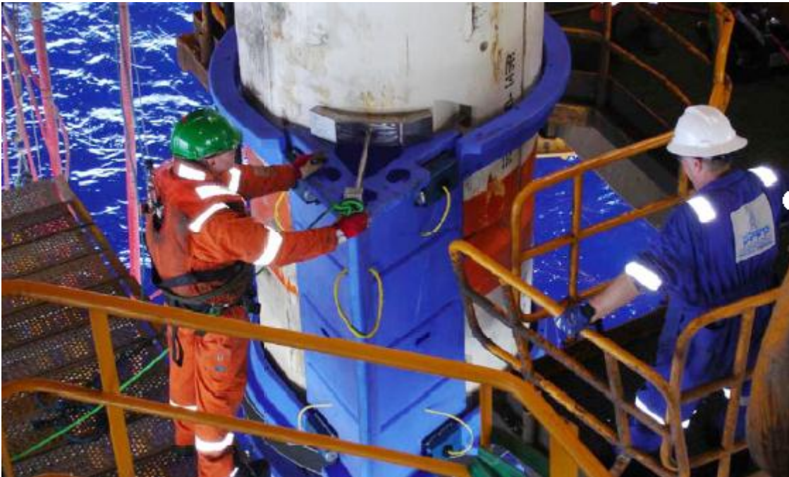
Figure 6.16 Fairing installation on drilling riser. Photo courtesy of VIV Solutions
