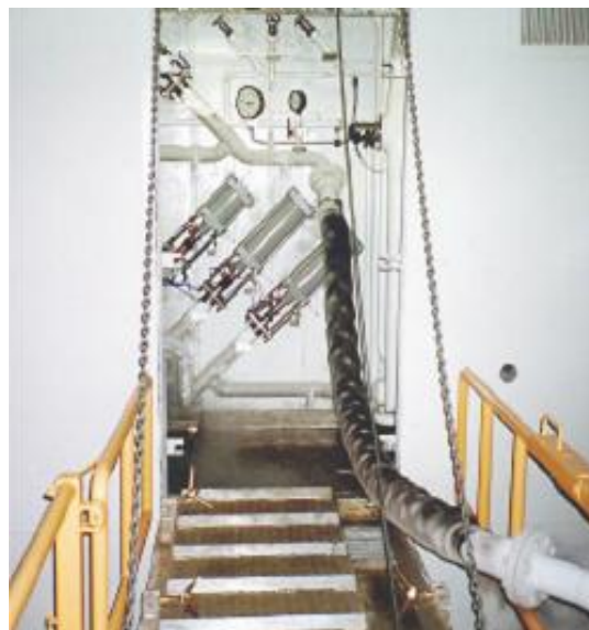
Figure 43. Bunkering of LNG from fuel truck to ferry. Courtesy MARINTEK.
