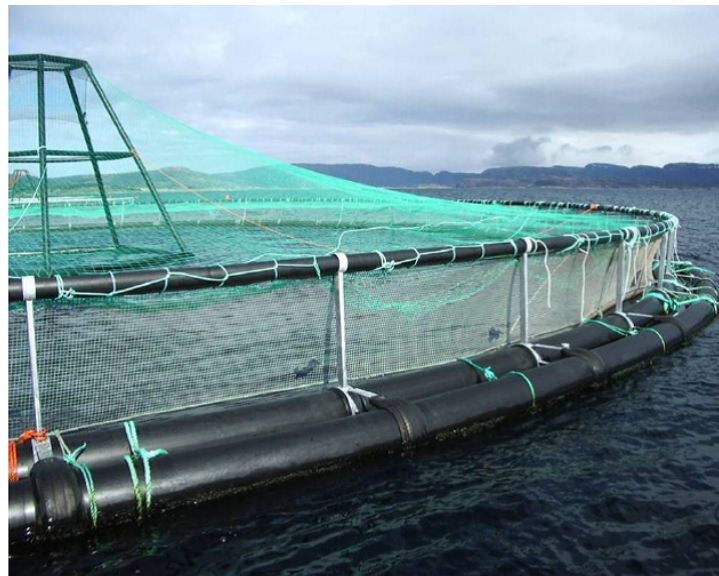
Figure 2.2: Floating fish farm with circular plastic collar consisting of two concentric rings. The photo is taken from [Faltinsen (2011)]. (Photo: SINTEF Fisheries and Aquaculture)
