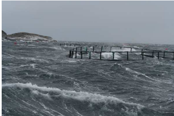
Figure 2.3: Fish farm with circular plastic collar in a storm in January 2006 in Flatanger, Norway. Elastic deformations of the floater are clearly seen. The photo is taken from [Kristiansen (2010)]. (Photo: Marius Dahle Olsen)
