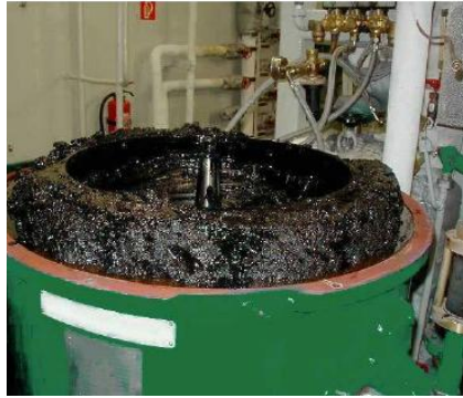
Figure 38: Clogged separator.
