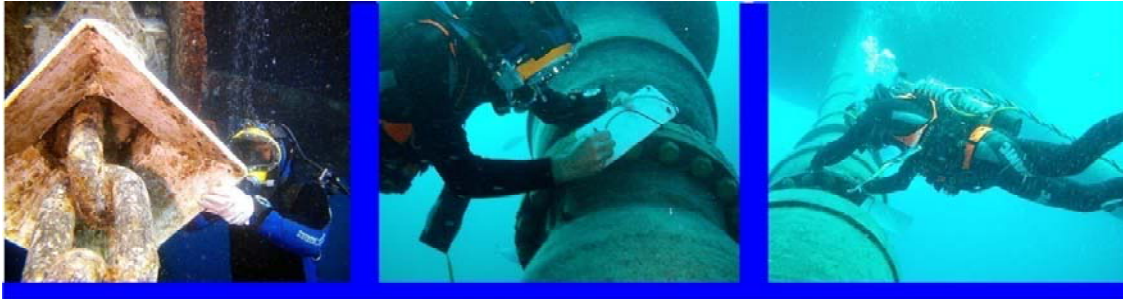
Figure 10 Divers carrying out inspection on pipelines and chain leg of a CALM buoy (Source: Tethys Plantgeria Ltd, Nigeria)
