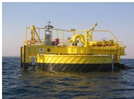
Figure 11 Calm buoy and offloading system (Source: Tethys Plantgeria Ltd, Nigeria)
