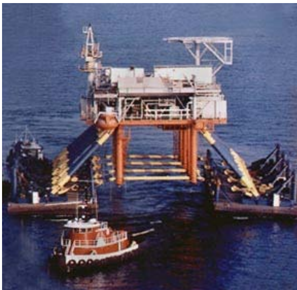
Figure 28: Topside lifted by the versatruss system, (Cash 1998)
