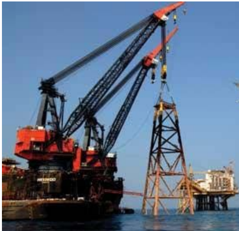
Figure 15: Hermod lifts a small jacket structure, (Terdre 2008)
