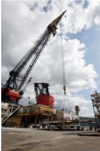
Figure 22: Hermod lifts the 37/22 heli deck ashore, (Sternhoff and Nordbakken 2009)
