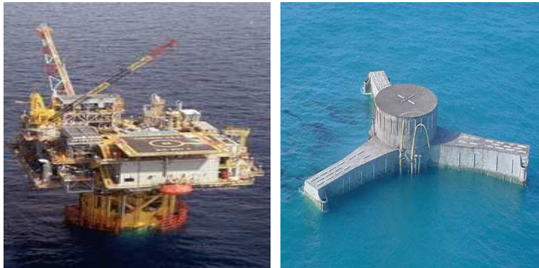
(a) Before Hurricane Rita
