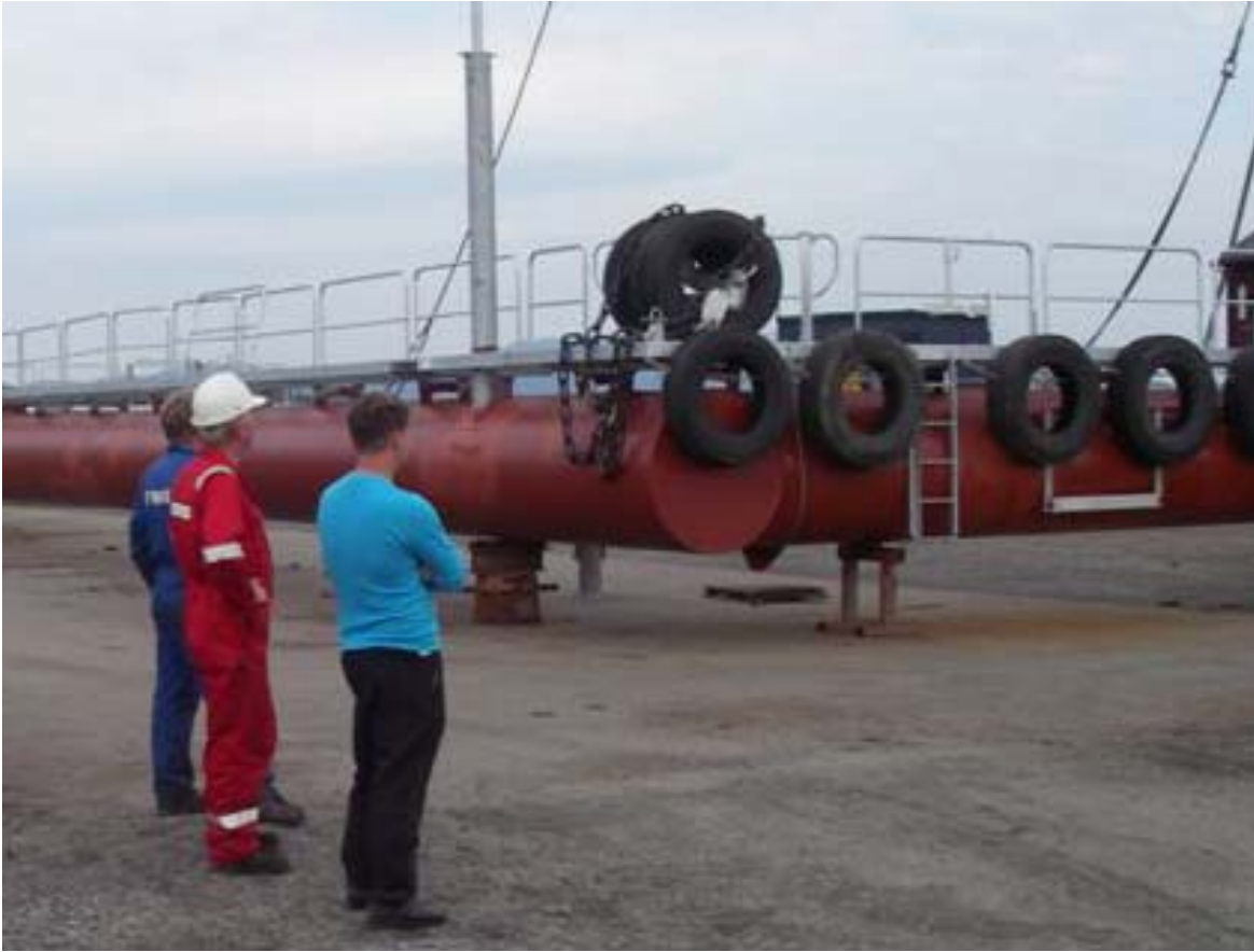
Figure 2.3: Fabrication of a steel floater (Photo: A. E. Lønning)
