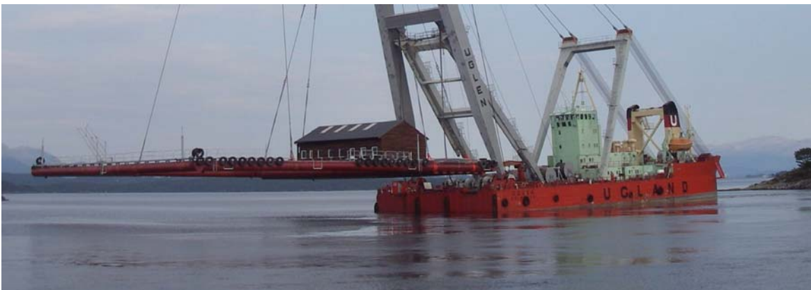
Figure 2.4: Installation of a steel floater (Photo: A. E. Lønning)
