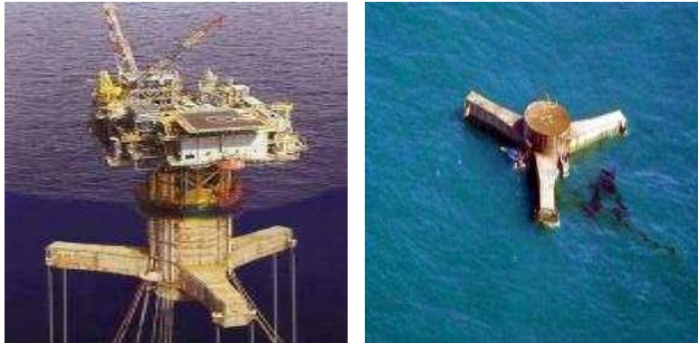
(a) Before the hurricane Rita. (b) Upside down following the hurricane Rita.
