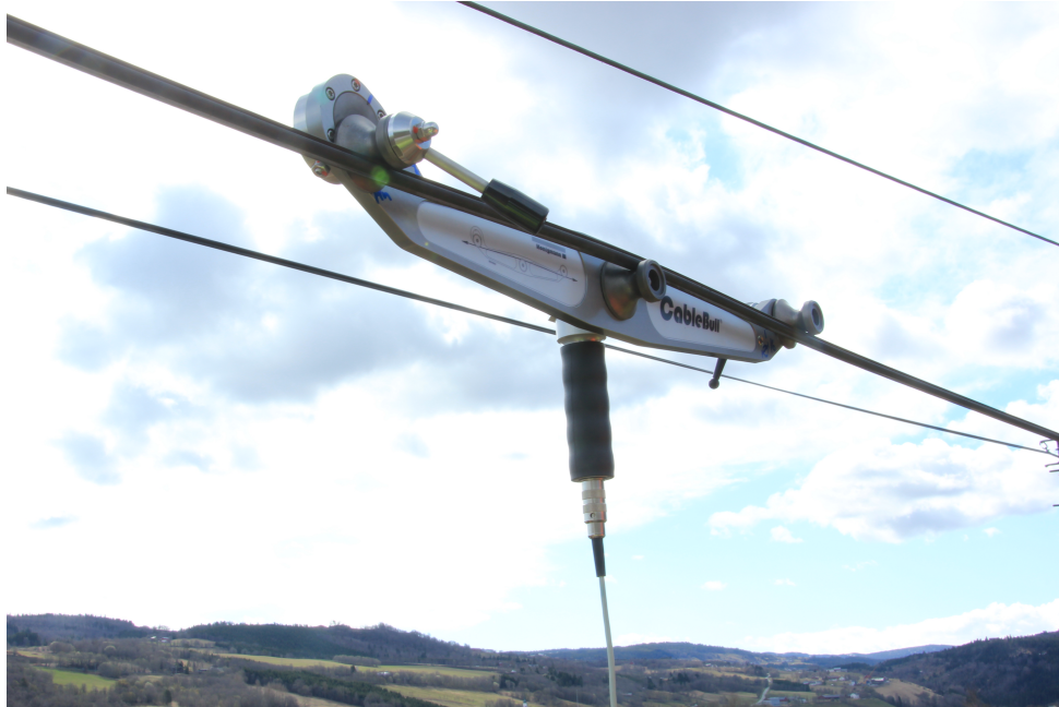
Figure 2.11: Device used to measure tension in the wires (Photo: Petter Røe Nåvik).
