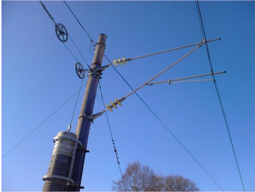
Figure 18 Picture of the tensioning equipment used at “Wire 152”
