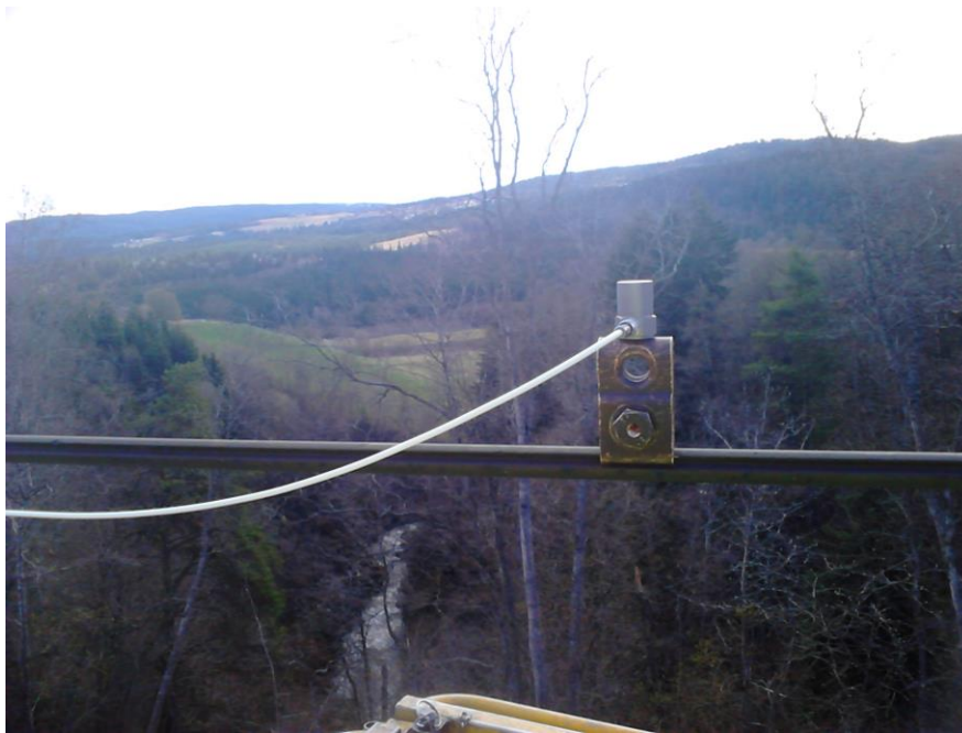
Figure 42 The fastening of the accelerometer the contact wire. The accelerometer is the grey thing on the top of the dropper clamp. The white cable sends the measured information to the computer.
