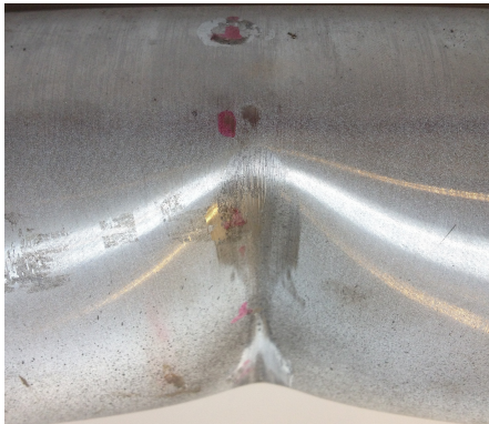
(c) Photo of pipe from Pipe 2.
