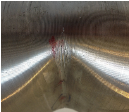
(a) Photo of pipe from Pipe 1.
