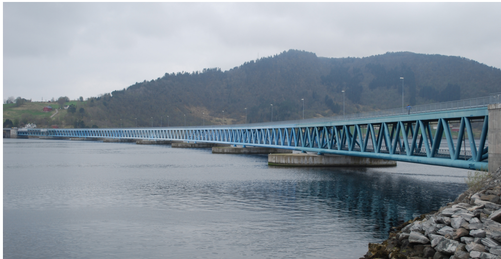
Figure 5.1: The Bersøysund Bridge. Photo: Cato Edvardsen.
