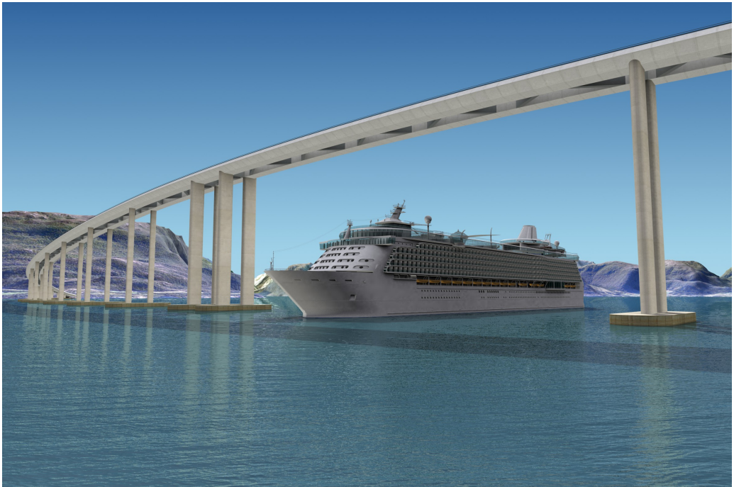
Figure 1.2: Concept model of floating bridge for the crossing of the Sognefjord. Illustration: Norwegian Public Roads Administration.
