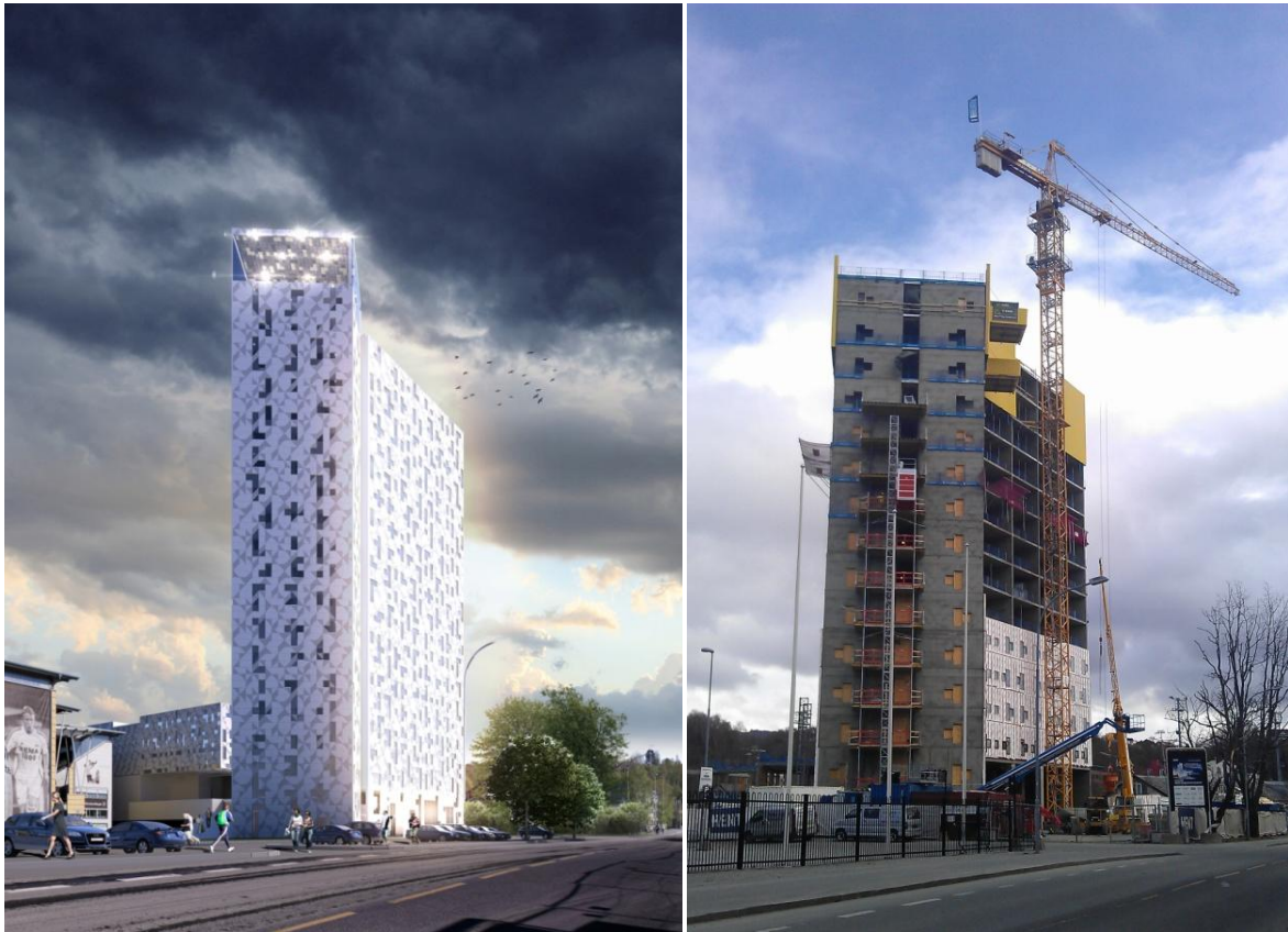
Figure 2.1: Left: Architectural sketch of Lerkendal Hotel. Right: Building under construction 24.04.2013
