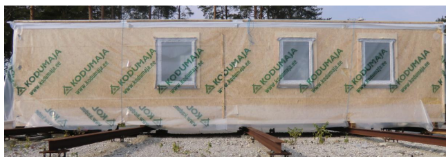
Long Exterior Wall
