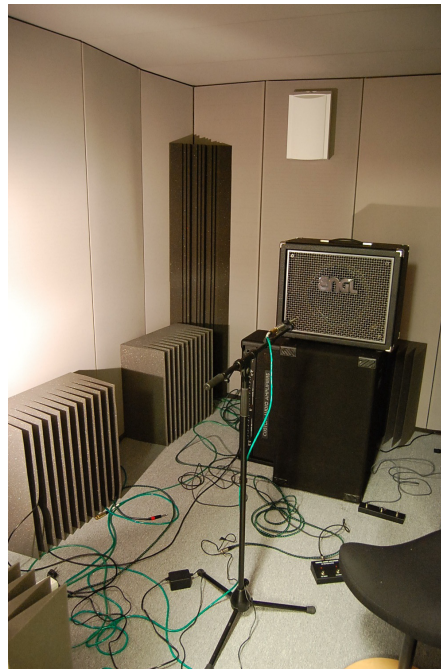
(b) Inside. The walls and ceiling are made of sound absorbers covered with a thin fabric. Each panel is slightly angled, to break up and deflect incoming sound waves. Additional sound absorbers were placed in the room to dampen it further.
