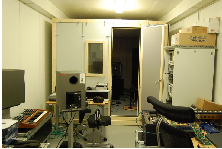
(a) Outside. The acoustic booth is a "room inside a room". All measuring equipment is operated from here.
