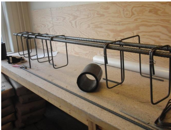
Figure 27: Reinforcement for beam A while being fixed
