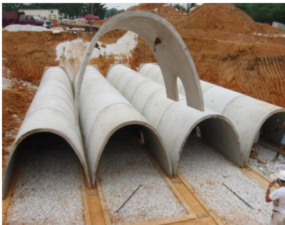
Figure 11: Storm water detention facility (Brodowski, et al., 2010)
