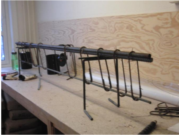
Figure 29: Reinforcement for beam B while being fixed
