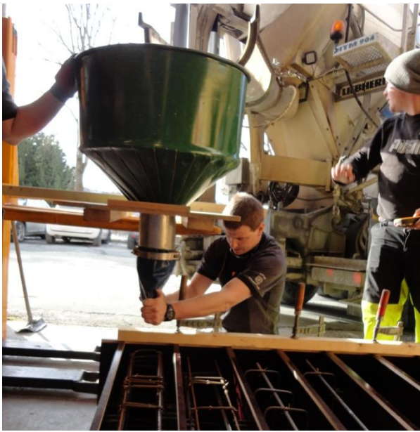
Figure 43: Hopper used for casting
