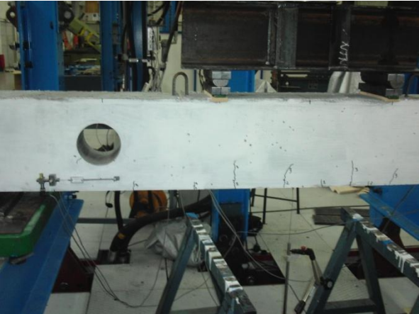
Figure 85: Initial cracking, beam C
