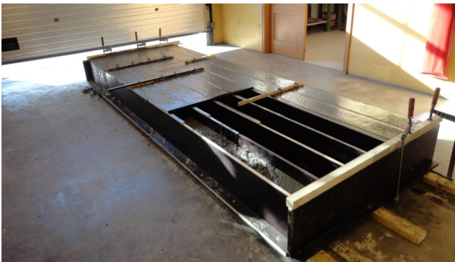
Figure 45: The beams after casting
