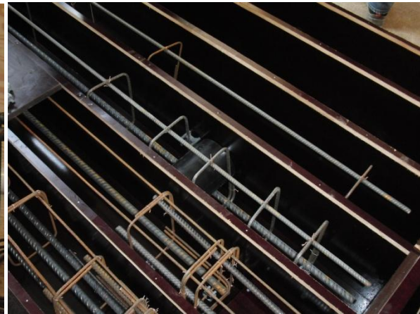
Figure 28: Reinforcement for beam A after being put into the mould
