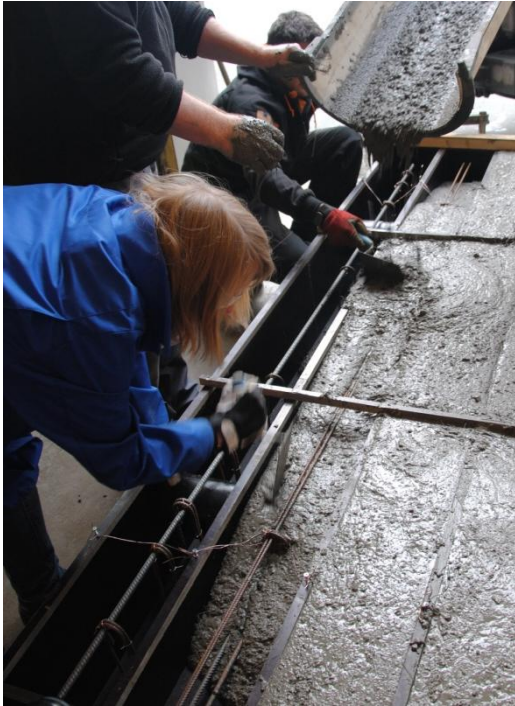
Figure 51: Casting of the SFRC beams
