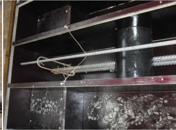
Figure 30: Reinforcement for beam C after being put into the mould
