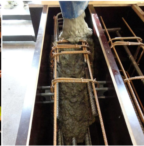
Figure 44: The casting process
