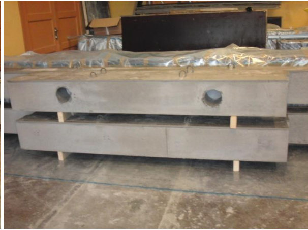
Figure 47: The beams piled for hardening
