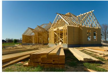
Figure 1.11: Light-frame construction, from [40]
