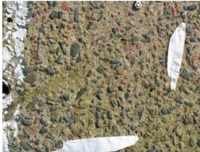
Figure 1 - 0.3 mm/yr ice abrasion on 90 MPa Confederation Bridge concrete after 8 years [15]
