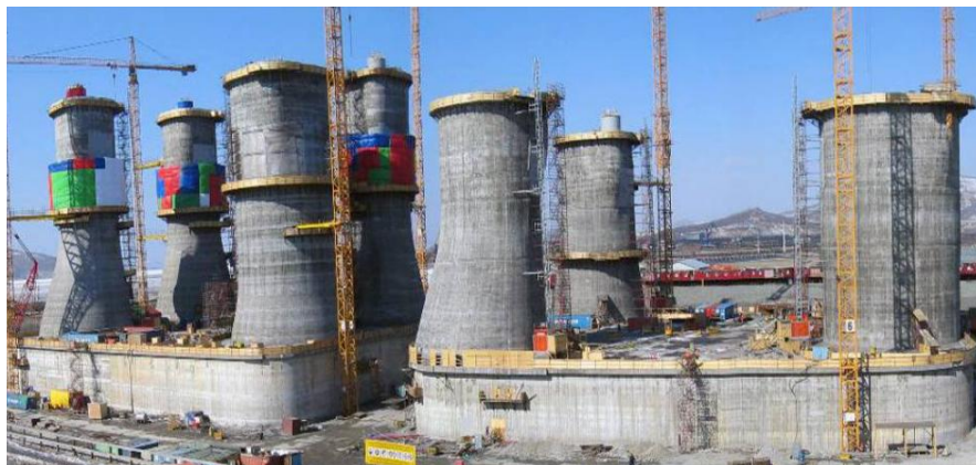
Figure 2 – Concrete structures placed in the Sea of Okhotsk 2004 and 2005, Fosså [19]
