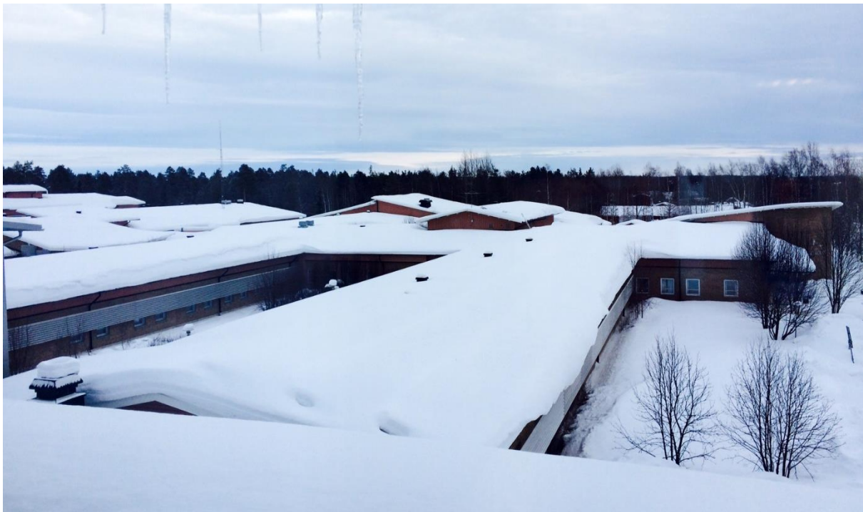
Figure 80 - Snow on the roof of the Acusticum. Roof A is the largest roof in the picture. Shot at 9 th of February 2015. Photo by Øystein Kleven.
