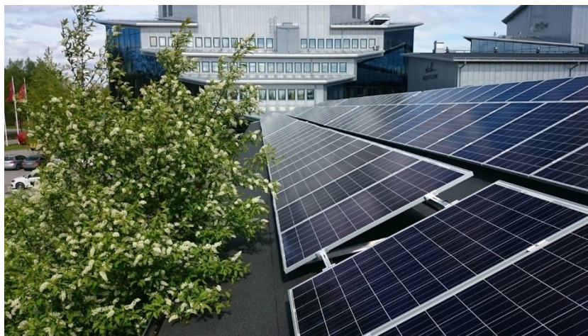
Figure 74 - Near shading from a tree at roof A. Photo by Eirik Oksavik Lockertsen.
