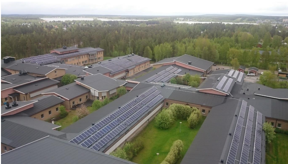
Figure 61 – The PV system at the Acusticum. Photo taken from the tower to the west. Photo by Eirik Oksavik Lockertsen.
