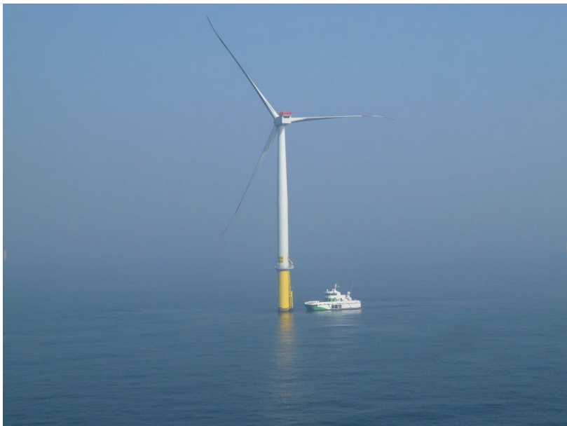
Figure 1.6: Umoe Ventus on the wind farm Borkum Riffgrund, by courtesy of Dong Energy.
