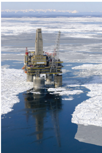
Figure 1.2: The Lunskeye-A platform in the Sakhalin II field (photo: Shell)
