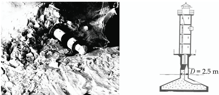
Figure 2.9: Nygrån lighthouse, collapsed in the winter 1968/69 (Bjerkaas 2006)
