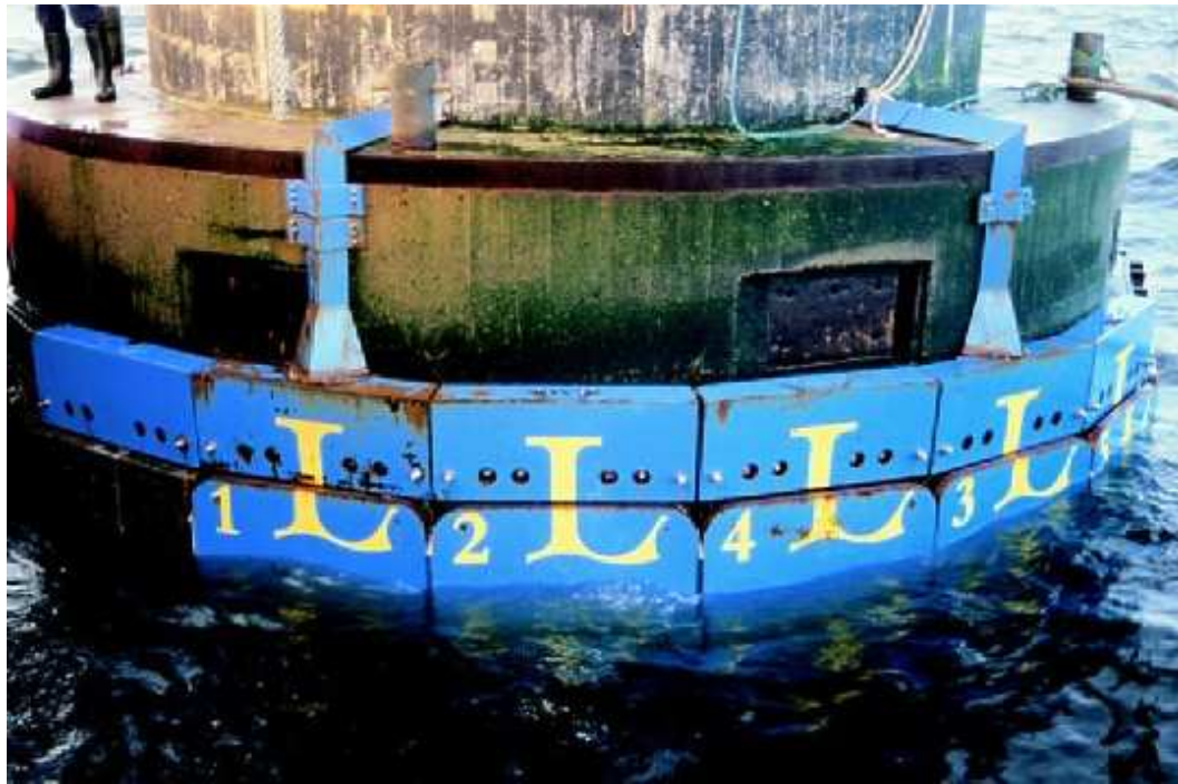
Figure 7.7: Panels installed at the lighthouse (Photo: Luleå University of Technology).
