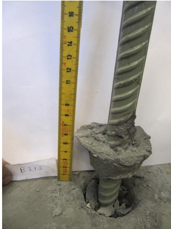
Figure 50 –The cohesion between the grout and the concrete block was weak and when the bolt was pulled out the grout was stuck on the bolt.
