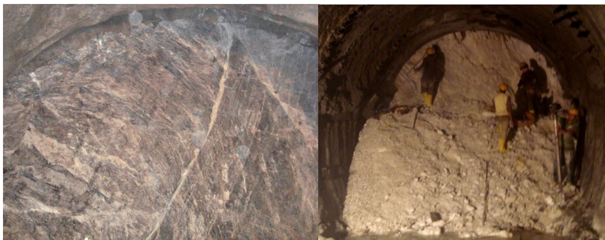
Figure 4-8: Rock mass condition at different chainage along headrace tunnel of CHEP
