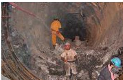
Figure 5-12: Evolution of the damage caused by squeezing between Chainage 12+750 and 12+850 (Hoek and Guevara, 2009a)
