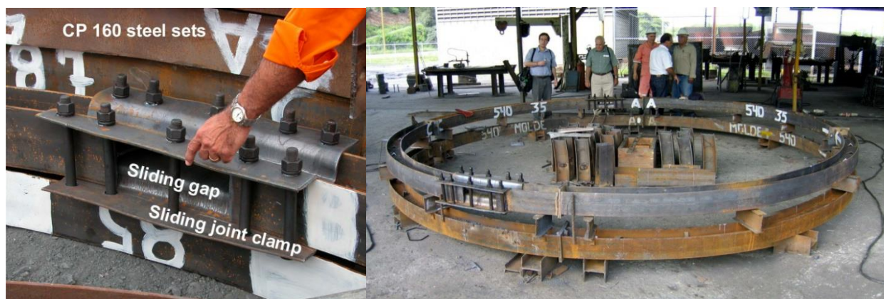
Figure 5-14: Details of one of the two sliding joints in the steel sets (left) and assembled steel set with two sliding joints (right) (Hoek and Guevara, 2009a)
