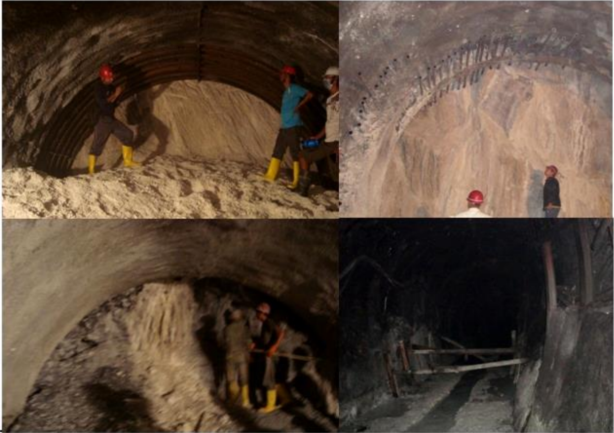
Figure 4-10: Several instances of tunnel excavation in CHEP at squeezing part
