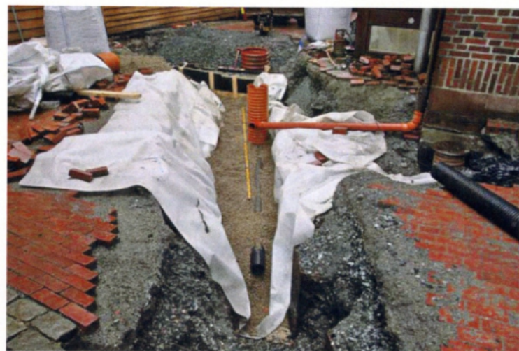
Figure 7.4: The underground infiltration structure at Bryggen (Christenson et al., 2012)
