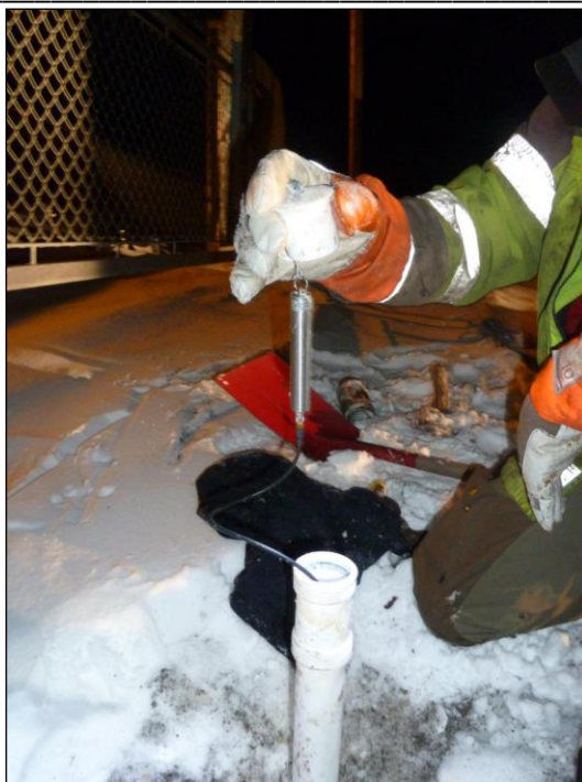
Figur 5-11: Thermistorstrengene settes ned i de 10 meter dype hullene.
